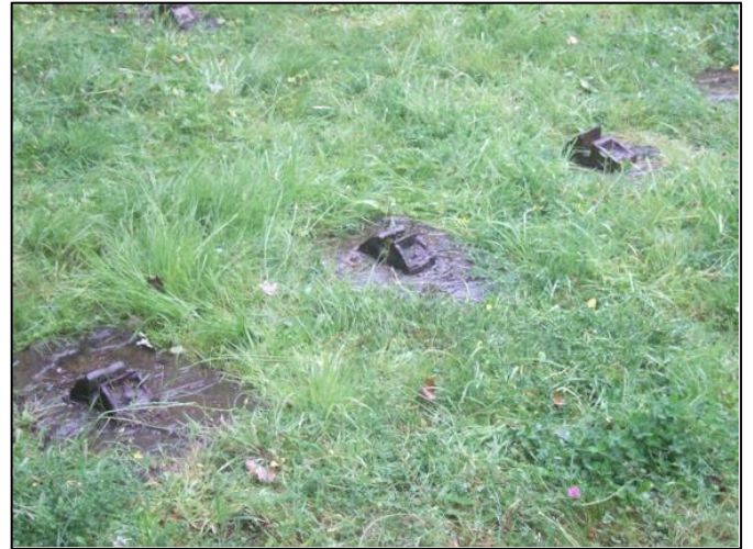
Dramway Rail Shoes & Stone Sleeper Blocks
