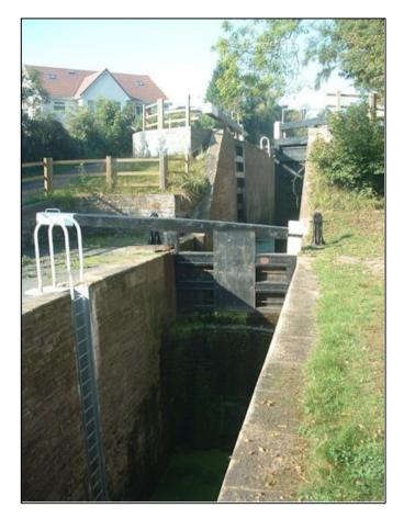
Fourteen Locks is a series of locks, also known as the Cefn Flight, on the Crumlin arm of the Monmouthshire Canal at Rogerstone in Newport. The flight of locks was completed in 1799 and raises the water level 50 metres in just 740 m. This is one of the steepest rises for a major run in the UK which, combined with the sheer number of locks, makes it one of the most significant in the country.
